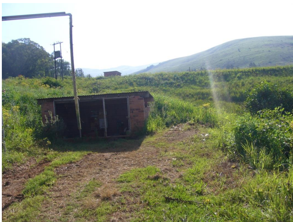
Figure 6: Mbangweni Embankment: Right Bank. Pump Station downstream of the dam
