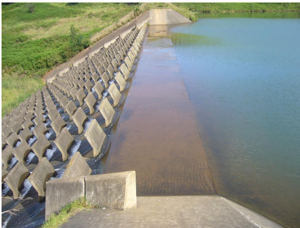
Figure 2: Baynesfield Dam: Concrete A-frame spillway with splitters
