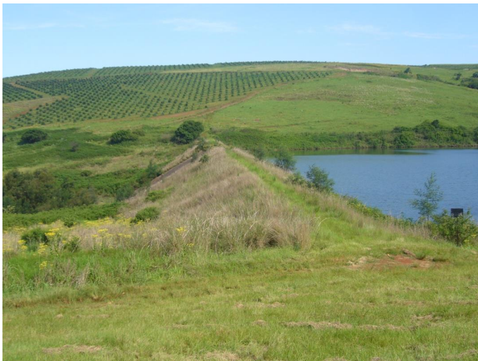
Figure 1: Baynesfield Dam: Dam viewed from the left bank
